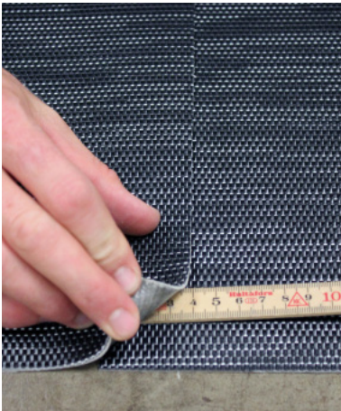
GRAPHIC 1. Overlap 2 sheets of flooring 4 cm and double cut.
